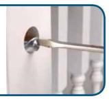
**7.** This will leave behind the end spindles, these can be simply lifted off their dowel pegs
