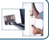
**2.** Remove the cover caps from the newel to expose fitting bolt for the handrail
