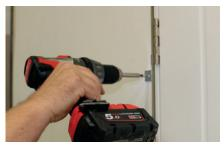
**STEP 3:** Screw the fixing brackets to the wall. Only screw them hand tight at this stage until step 4 is complete.
