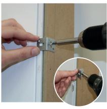
**STEP 1:** Unscrew all fixing brackets, reverse them and re-fit ready to offer the doorset to the opening.
