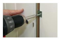
**STEP 5:** Fully tighten the screws in the fixing brackets.
