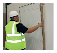
**STEP 2:** Offer up the doorset into the opening, use packers on the edges of the doorset if required. To increase floor covering clearance, packers may be positioned under each jamb.
