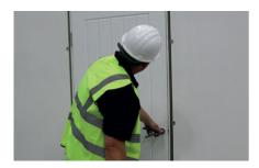
STEP 11: Test the door closes into the frame correctly, ensuring that the door does not bind or catch in the frame.
