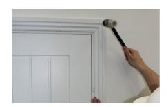
STEP 19: Add the final vertical piece of architrave, using a soft mallet if required. Making sure the architrave is level. Final fix using pins.
