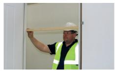
**STEP 9:** Using the timber packing bar removed in step 6, position onto the frame and slide down from top to bottom checking for tightness or excessive gaps.
