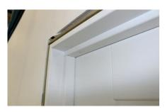
**STEP 14:** Fix the two vertical door stops in position, using an appropriate grab adhesive and pins.
