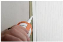
STEP 17: Apply an appropriate grab adhesive to the groove in the lining that the architrave will be positioned in.
