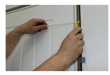
**STEP 6:** Now the doorset is in place, remove the plastic banding and the timber packing bar.
