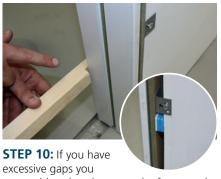
must add packers between the frame and the opening equally at either side.
