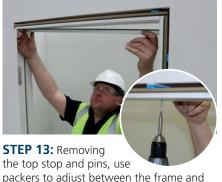
packers to adjust between the frame and the opening and fix in the centre. Using grab adhesive or pins refit the top stop.
