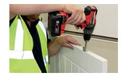
**STEP 7:** Unscrew and remove the metal transport bracket at the top of the doorset.
