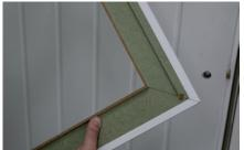
STEP 16: Using the Hoffmann Key provided assemble both pieces of the architrave together.
