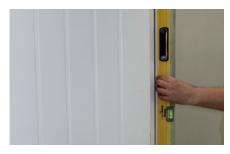
**STEP 8:** Using a spirit level, make sure the door and the frame is plumb and square.
