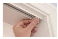
Offer the door back up to the opening, folding the doors and engaging the top pin pivot and the roller guide into the track. You may need someone to help you with this.
