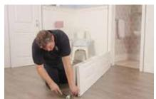
Vertical adjustment can also be made by screwing the bottom pivot up or down.
