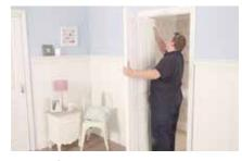
You can adjust the top pivot in the track to set the edge gap, to ensure the door opens correctly.
