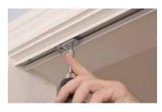
**8.** Add the spring closer that will create tension to hold the door closed, and also soften the door closing operation.
