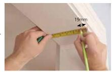
2. To determine which way to position the track, you will need to decide which way you want the door to fold - either to the left or the right. In this instruction we are fitting a left hand fold door, so the pivot
