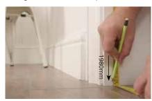
**4a.** Measure and mark 19mm from the inside edge of the frame backwards to position the bottom pivot bracket.
