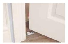
**5a.** Offer the door up to the opening to identify where to position the top pin pivot and top roller guide.
