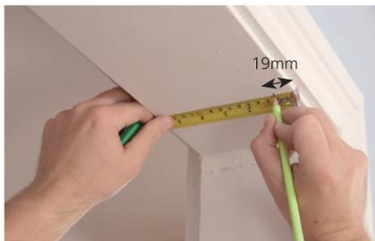
2. To determine which way to position the track, you will need to decide which way you want the door to fold - either to the left or the right. In this instruction we are fitting a left hand fold door, so the pivot bracket should be positioned to the left. This will be on the opposite side if a right hand fold is required.
