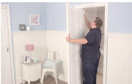
7. Slot the bottom pivot into the bottom pivot bracket.
