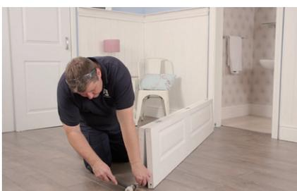
You can adjust the top pivot in the track to set the edge gap, to ensure the door opens correctly.
