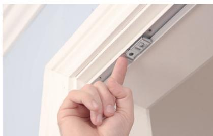
Ensure the track is level and central within the door frame, use the screw holes to mark and pilot drill the screw positions.
