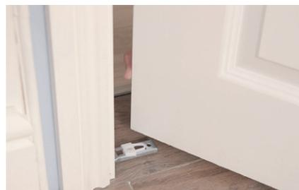
\*Refer to the diagram opposite for hardware locations. Slot the pivots loosely into the pre-drilled holes.
