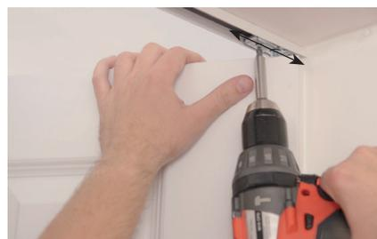
6. Unscrew and release the top pivot in the top metal track.
