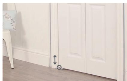
Offer the door back up to the opening, folding the doors and engaging the top pin pivot and the roller guide into the track. You may need someone to help you with this.
