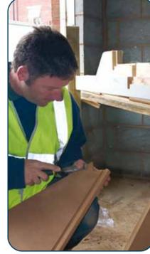
Make sure the profiling of nosing is correct to fit in newel housing. (If not done correctly it can force newel post out of level).
