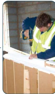
Remove newel. Using 10mm drill bit, drill through bore hole on newel post onto tenon of string by offsetting hole 2mm closer to shoulder of tenon.
