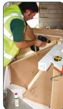
Make sure glue blocks are glued on all loose risers. Screw and glue winder treads to newel posts making sure at all times the newel is square to the last tread and loose wall string is square to main string.
