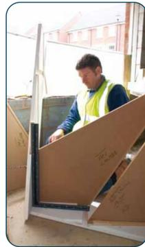
Again making sure profiling is correct to fit in trenching nosing on wall string.
