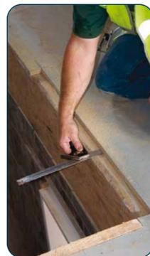
It is advisable to leave a gap of 2-3mm between landing boards and nosing to stop any chance of forcing the newel out of level.
