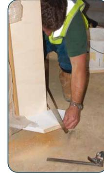
then on both top and bottom string cut for depth of skirting board.
