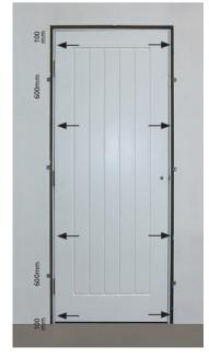
= Fixing points through the door stop groove in the lining.
