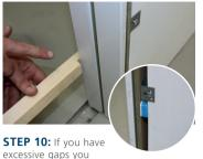
excessive gaps you must add packers between the frame and the opening equally at either side.
