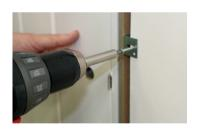
**STEP 5:** Fully tighten the screws in the fixing brackets.
