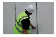
STEP 11: Test the door closes into the frame correctly, ensuring that the door does not bind or catch in the frame.
