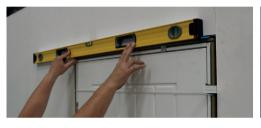
**STEP 4:** Using a spirit level, check the doorset is positioned square in the opening at all edges, pack where necessary.
