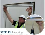
the top stop and pins, use packers to adjust between the frame and the opening and fix in the centre. Using grab adhesive or pins refit the top stop.
