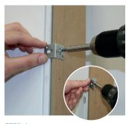
**STEP 1:** Unscrew all fixing brackets, reverse them and re-fit ready to offer the doorset to the opening.
