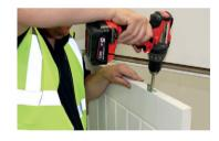
**STEP 7:** Unscrew and remove the metal transport bracket at the top of the doorset.
